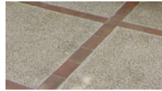
Decorative cement & bricks
