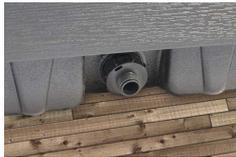
**Step 1:** Remove the drain cap.
