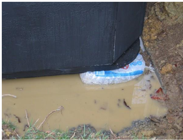
Figure 8. Swim Spa and Exercise Pool Position in Excavation on Ice Bag
