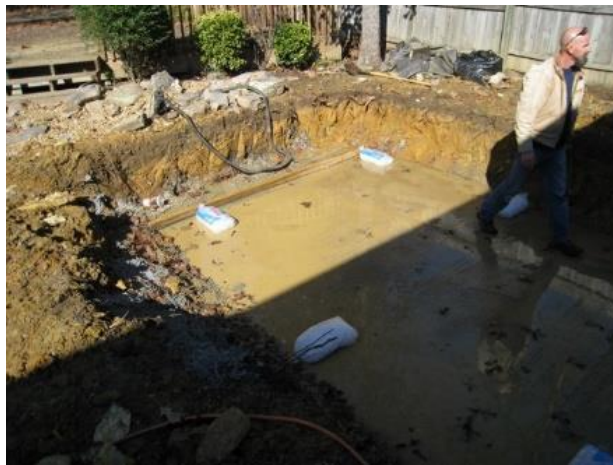
Figure 7. Ice Bag Positioning in Excavation
